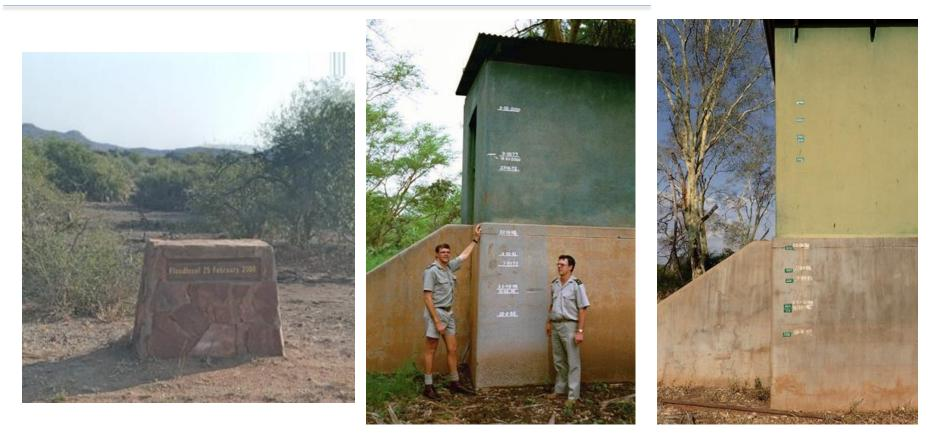
Marked historic floods levels: left) (February 2000) - on beacons on the tar road crossing the Luvuvhu River, Middle) marked on a wall at the Theba Pump House between 1958 and 2000 - date unknown, Right) includes the 2013 flood that is the second highest recorded after 2000 (photograph October 2022)
